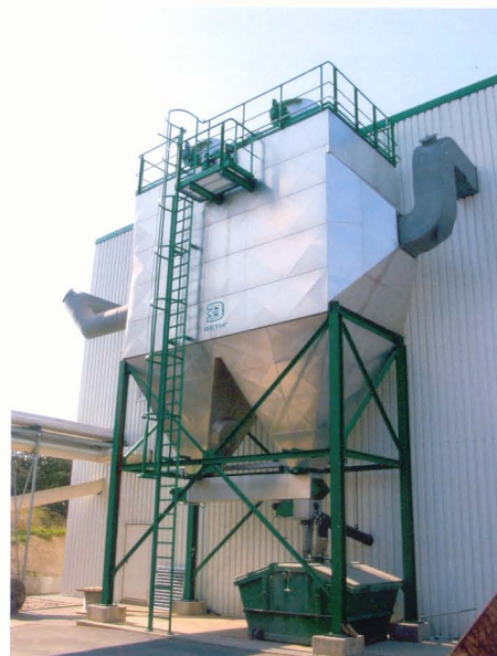
BETH standard electrostatic precipitator Sewage sludge incineration, 45,000 Bm 3 /h < 20 mg/Nm 3 dry at 230° Celsius
