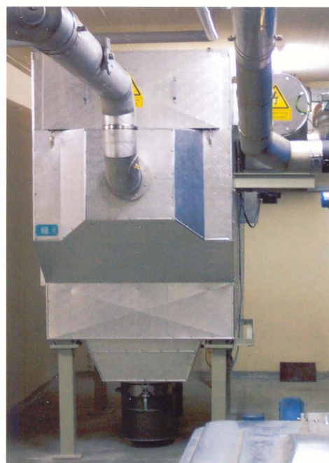
BETH mini electrostatic precipitator Biomass incineration system, 3,080 m 3 /h < 40 mg /Nm 3 dry at 300° Celsius
