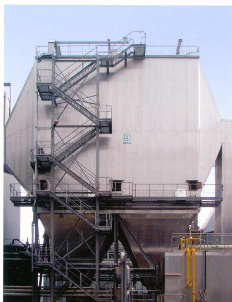
BETH industrial electrostatic precipitator Biomass boiler system, 435,000 Bm 3 /h < 20 mg /Nm 3 dry at 400° Celsius
